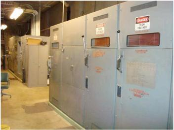
The high voltage distribution center was installed in the 80's. It provides the incoming MidAmerican Energy interface to the campus. At this point Drake Facilities is responsible for all the high voltage and secondary (user) voltage on campus. By purchasing power at the primary voltage level (13,200 volts) Drake can cut their electrical energy bill by 40%. The trade off is Drake absorbs the cost of the equipment, maintenance and depreciation.
