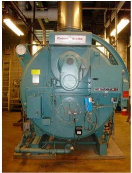
This is the same model of boiler but in the 350 HP size. We use this boiler in the summer to give the 800 Cleaver Brooks boilers a break for maintenance, and to save energy. Steam is still needed to cook and make domestic hot water as well as to keep the system hot for preservation of the underground piping.
