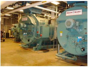
These are two 800 HP Cleaver Brooks boilers which make 50 pound steam to heat the entire central campus. One boiler will heat campus up to 0 degree days before the other is needed. These boilers also provide steam to heat domestic water, to cook and humidify some buildings on campus. Previous to the plant remodel the same job was done with 1200-2000 HP boilers.
