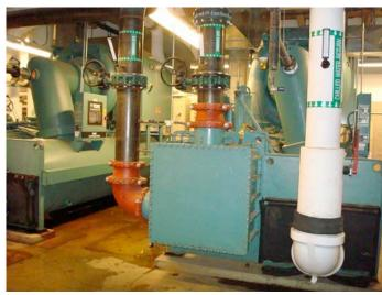
This is the 750 Ton York chiller with variable frequency drive. The variable frequency drive runs the chiller at only the speed necessary to do the job, which is to make 42 degree water. This is a big energy savings over the traditional chiller which is either on or off.
